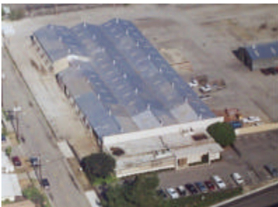
50,000 Sq.Ft. Manufacturing Facility Los Angeles Lighting Mfg. Co. El Monte, CA
